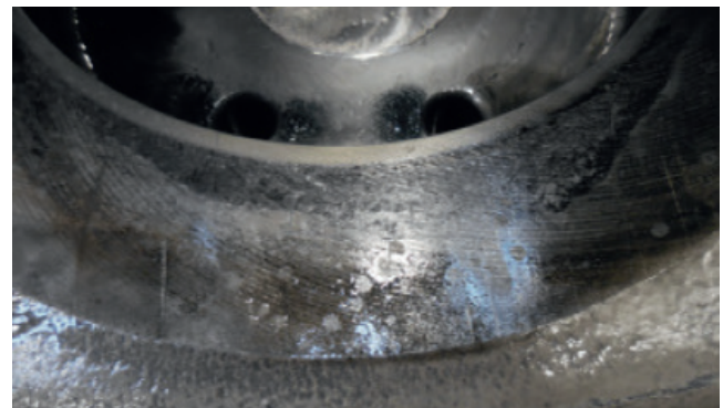
Gearbox with surface damage due to micro-friction
