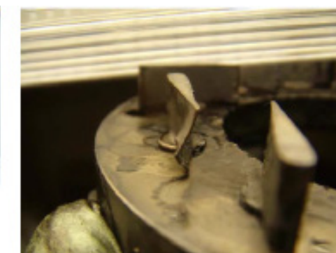
Damaged nozzle blades
