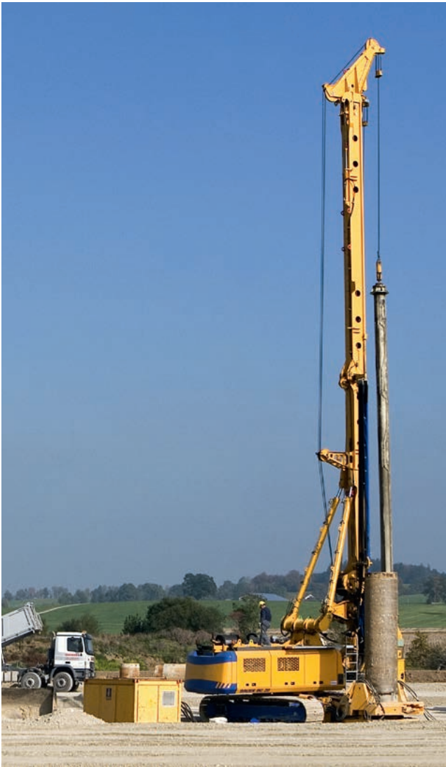
Pile-driving and drilling machine
